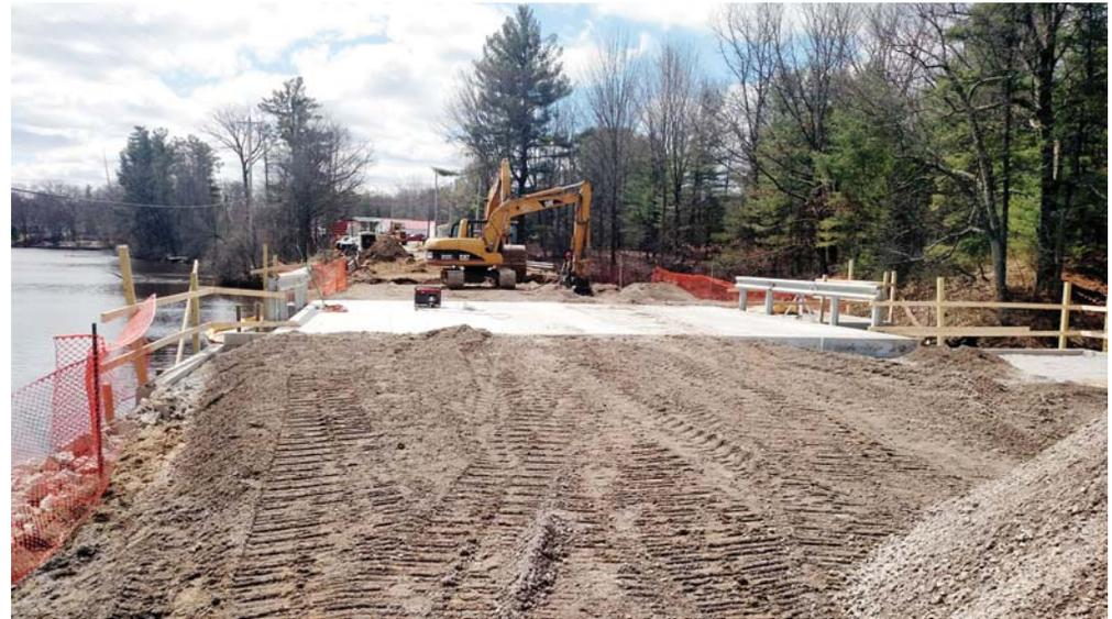
This bridge structure type is the first of its kind to be constructed in the Great Lakes Bay Region and the second in the State of Michigan. The bridge is a GRS-IBS (Geosynthetic Reinforced Soil-Integrated Bridge System) structure that has a 22' span and 7' plus headroom for smaller boat traffic. High strength concrete slabs were used for the bridge deck.
