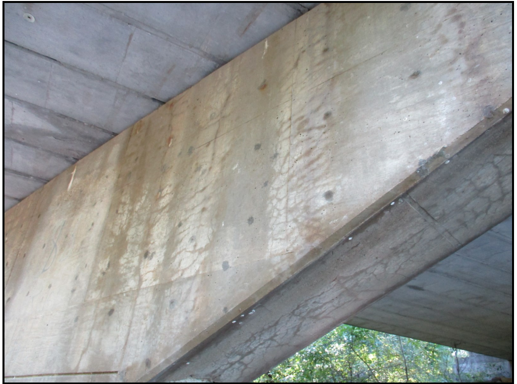
Hairline cracking throughout pier
