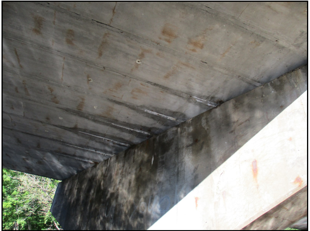
Leakage in grout joints at pier
