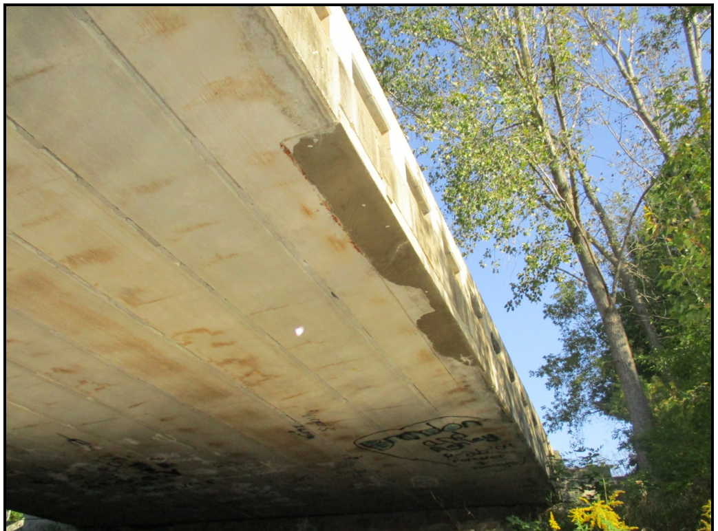
Patched area on east fascia beam, span 3S
