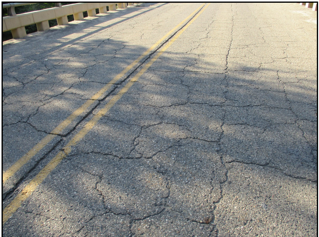
Cracking throughout HMA surface
