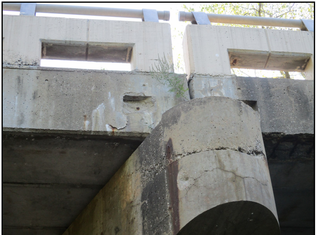
Spalled grout in post tension pockets on west fascia
