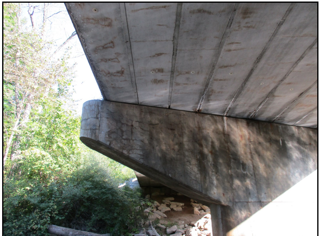
Map cracks in north pier
