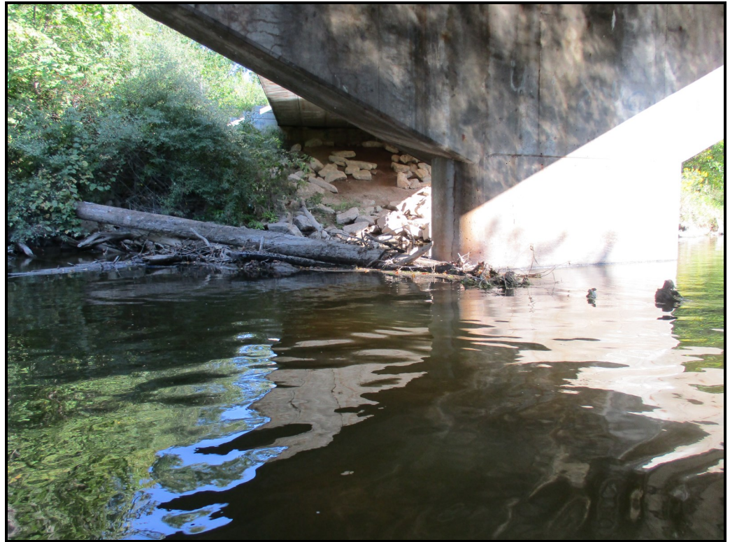
Debris stuck on north pier
