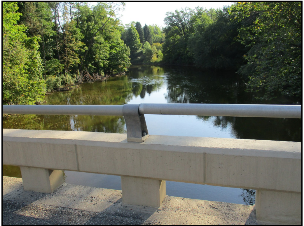
Loose tube on east rail
