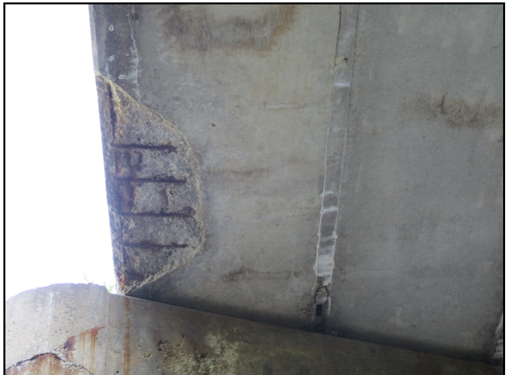
Span 1S, beam 1W, spall on bottom at pier
