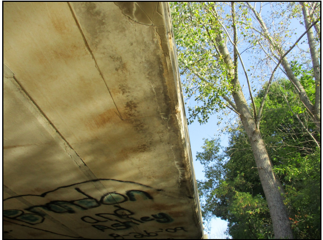
Leaching crack on east fascia beam, span 3S
