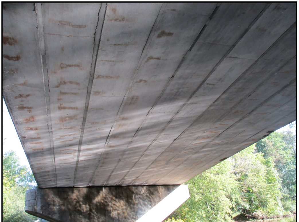
Center span box beams
