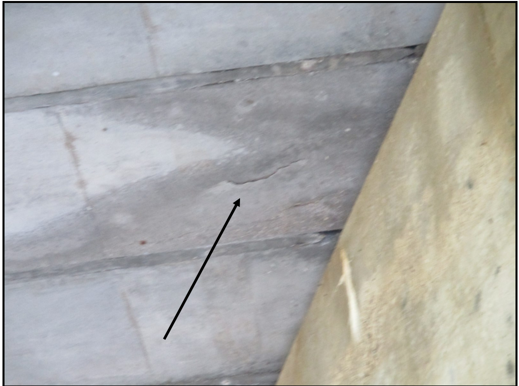
Delamination on bottom of beam 6W, span 2S
