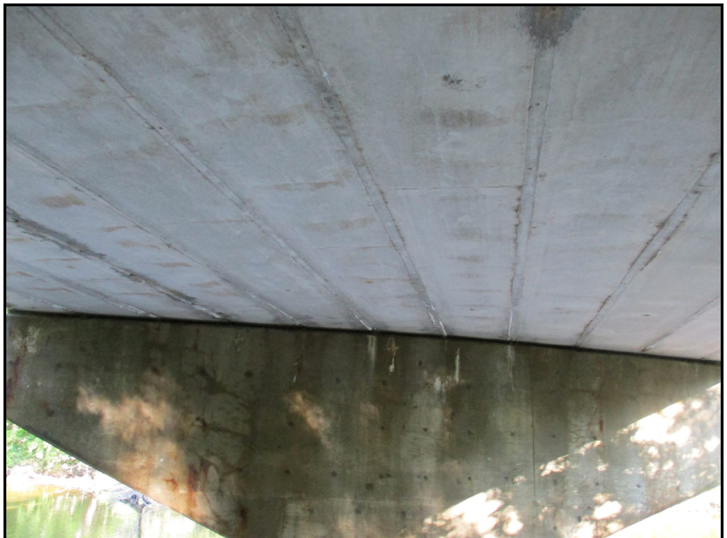
Bottom of box beams
