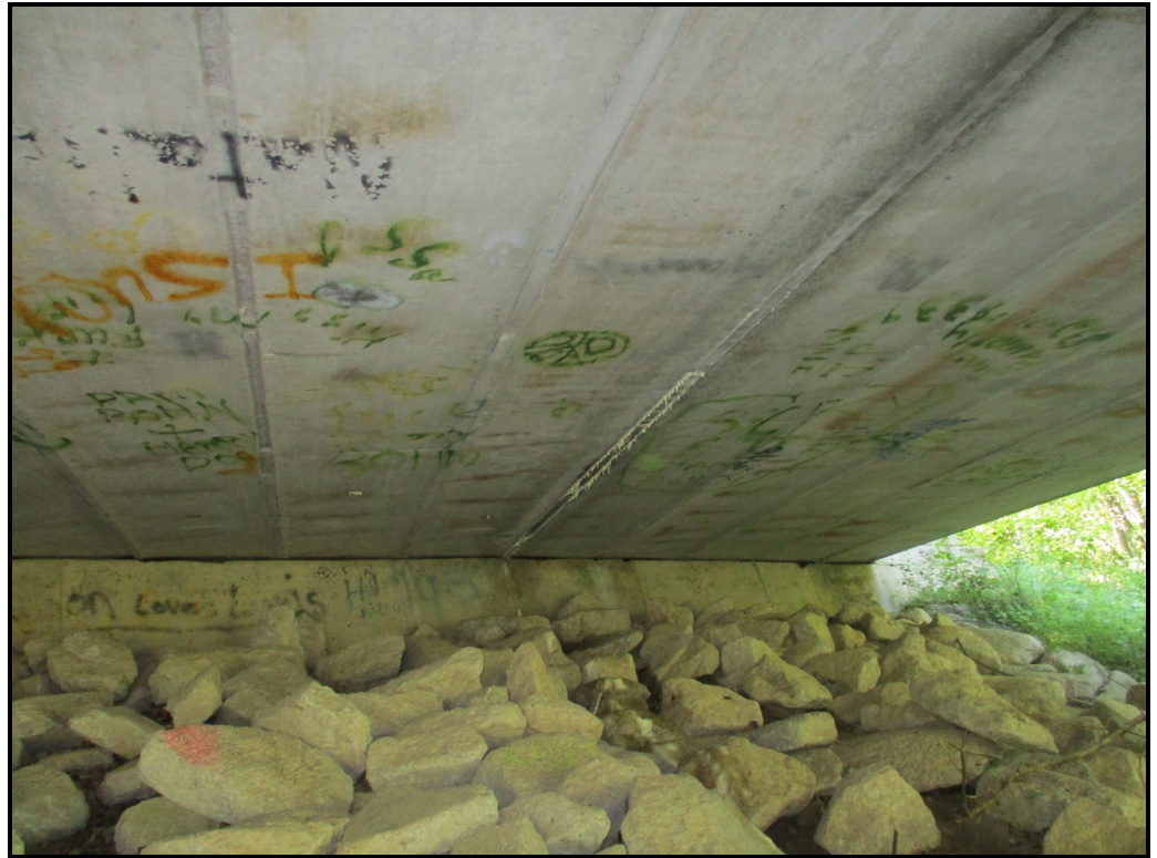
Leakage along grout joint
