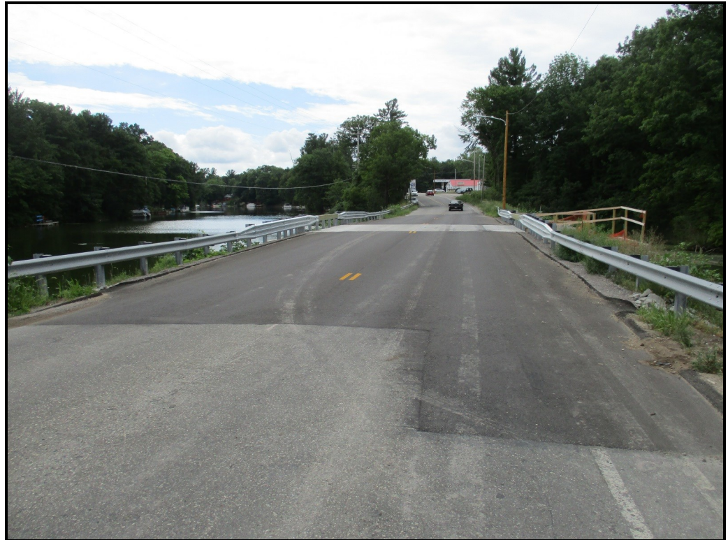
Road and bridge section facing south
