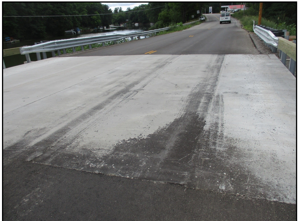
Top of precast concrete slabs
