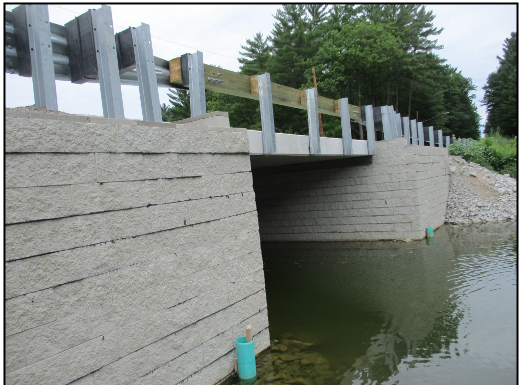
East elevation of bridge
