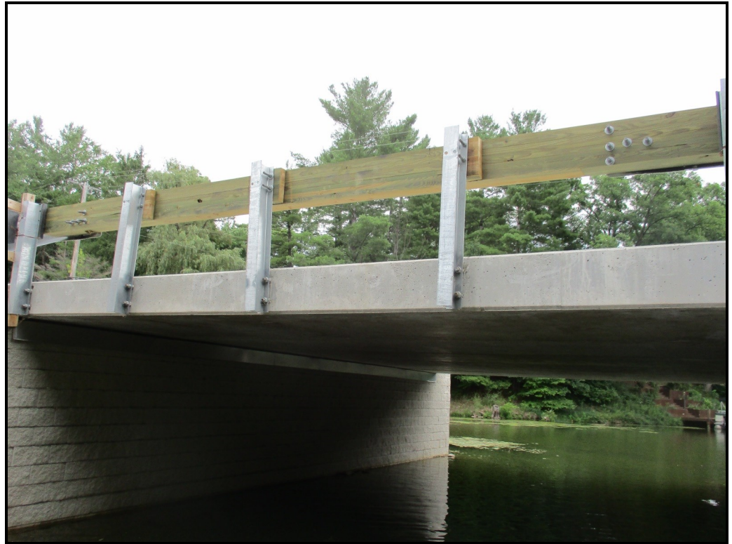
West elevation of bridge
