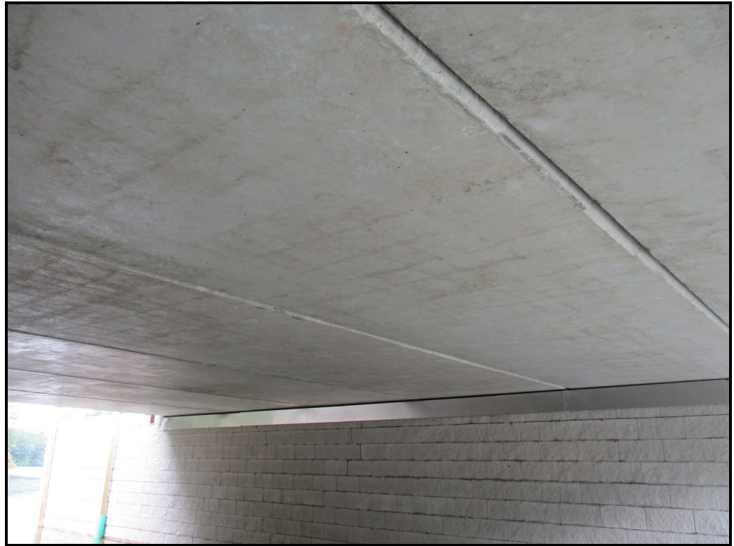
Bottom of precast concrete slabs
