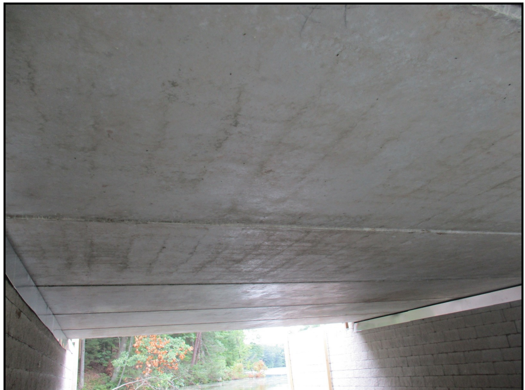
Bottom of precast concrete slabs
