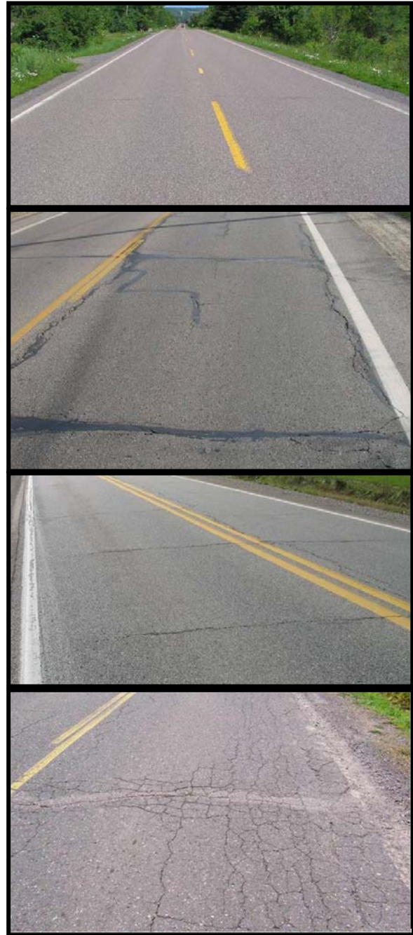
Figure 2: Top image, right – PASER 8 road that is considered “good” by the TAMC exhibit only minor defects. Second image, right – PASER 5 road that is considered “fair” by the TAMC. Exhibiting structural soundness but could benefit from CPM. Third image, right – PASER 6 road that is considered “fair” by the TAMC. Bottom image, right – PASER 2 road that is considered “poor” by the TAMC exhibiting significant structural distress.
