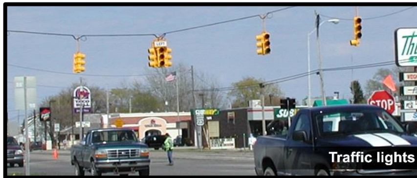
Figure D-1: Example of traffic signals
