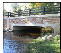
Figure 4: Three-sided box bridge
