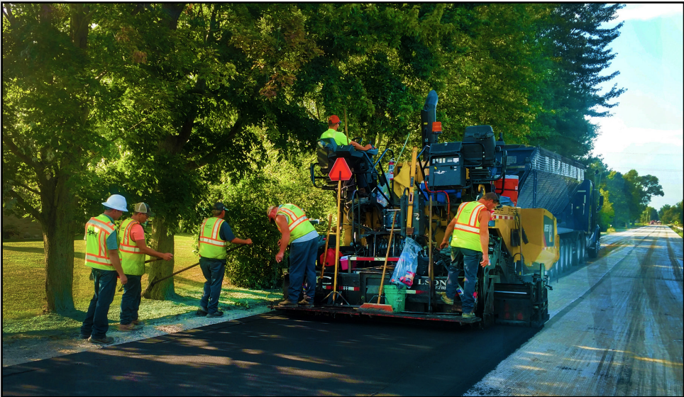
Crews apply asphalt made from recycled plastic bags, increasing the life of the road.
